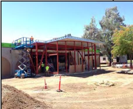
Board Room structural steel is complete.
