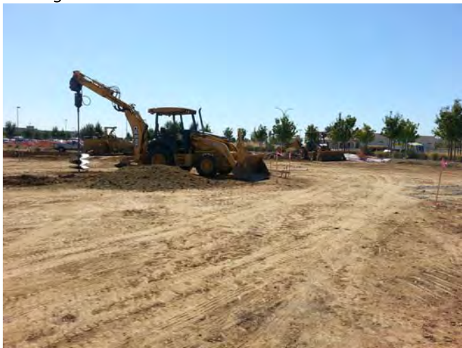
Parking Lot in construction
